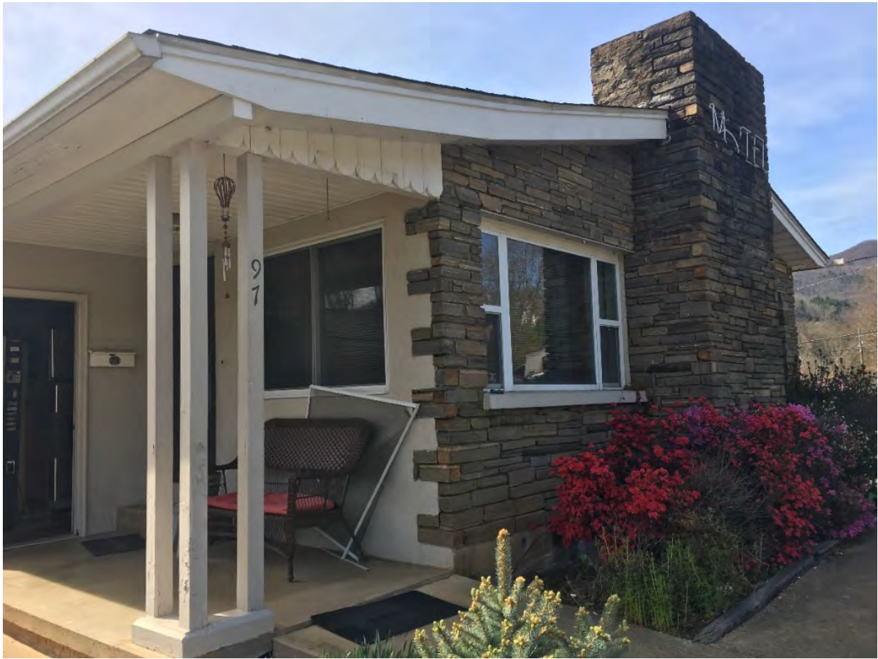
FIGURE 13: Current photo of the east façade of the office facing northwest
