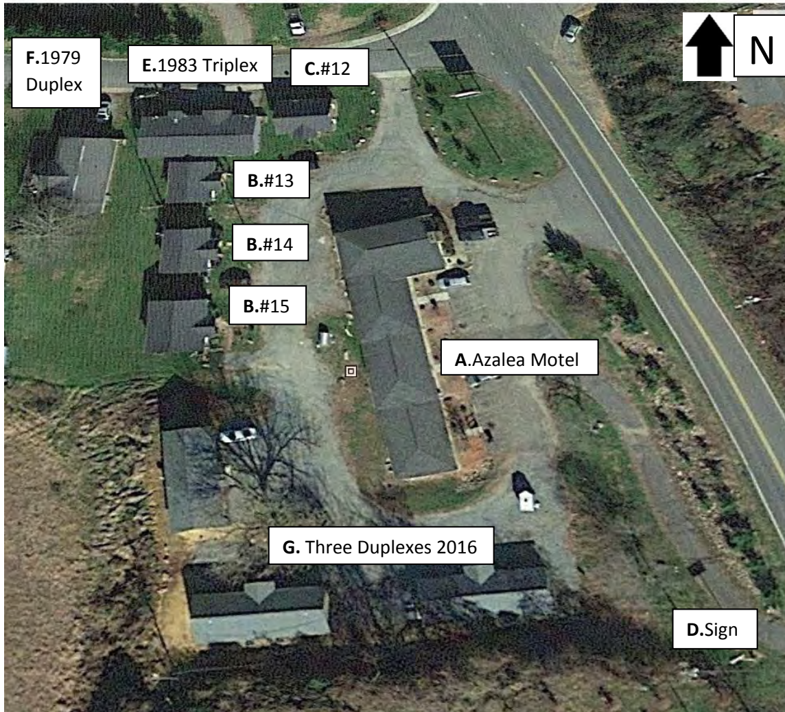
FIGURE 4: Google Earth Aerial photo with locations of structures
