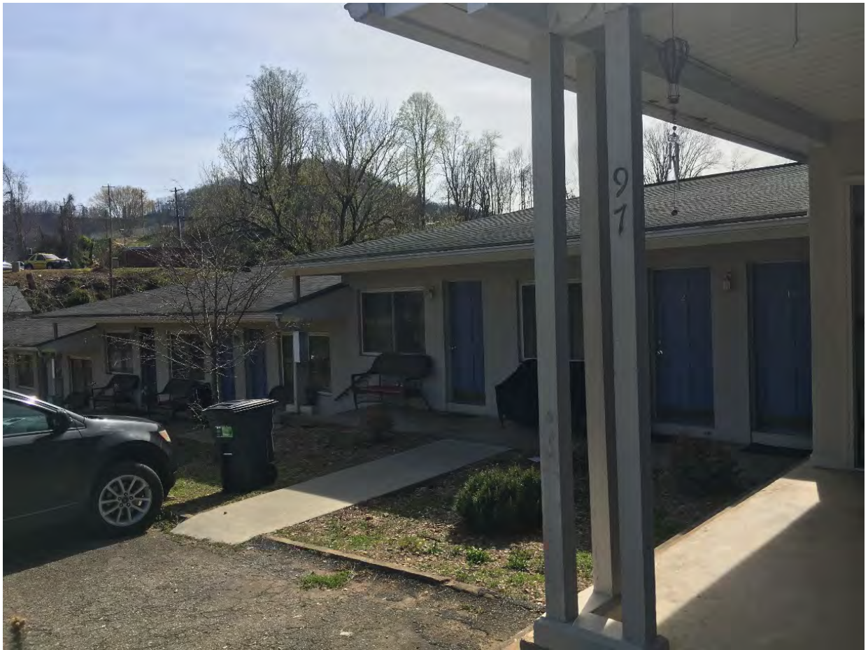
FIGURE 15: Current photo of the east façade of the motel facing southwest
