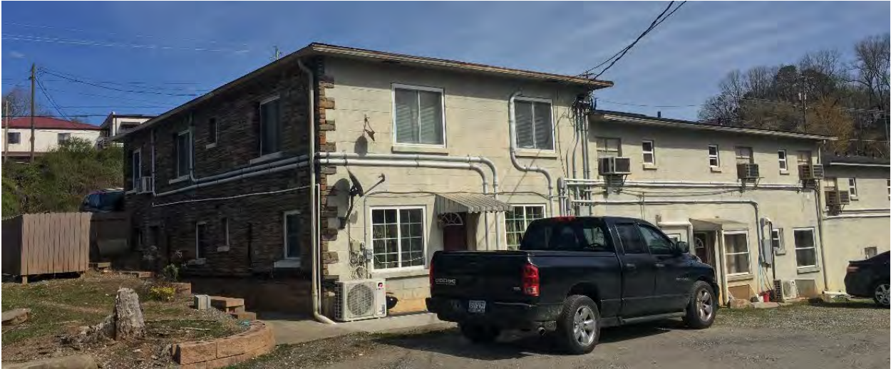
FIGURE 18: Current photo of the west façade of the office facing southeast
