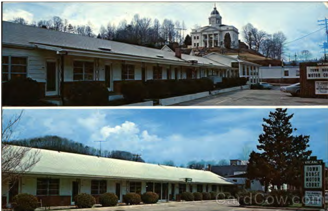
FIGURE 42: Blue Ridge Inn (Town House Motor Court), postcard views, ca. 1959 (source: https://www.cardcow.com/480914/town-house-motor-court-sylva/ )
