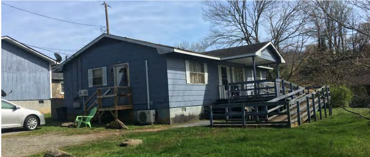
FIGURE 29: Current photo of the north elevation and façade of the duplex facing south
