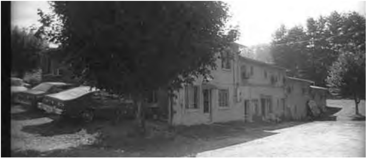
FIGURE 17: 1989 survey photo of the west façade of the motel facing southeast
