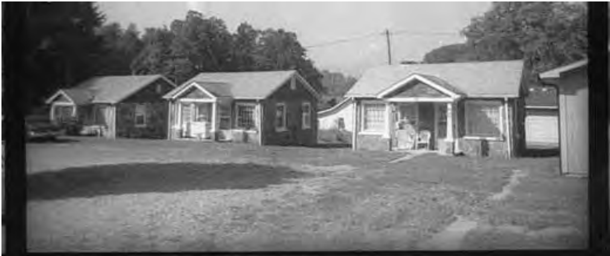
FIGURE 21: 1989 survey photo of the façade of the #15, #14, and #13 cottages facing west
