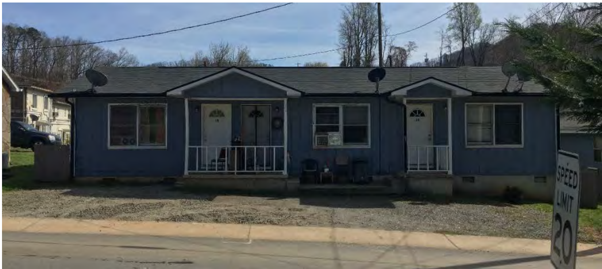
FIGURE 28: Current photo of the façade of the triplex, facing south
