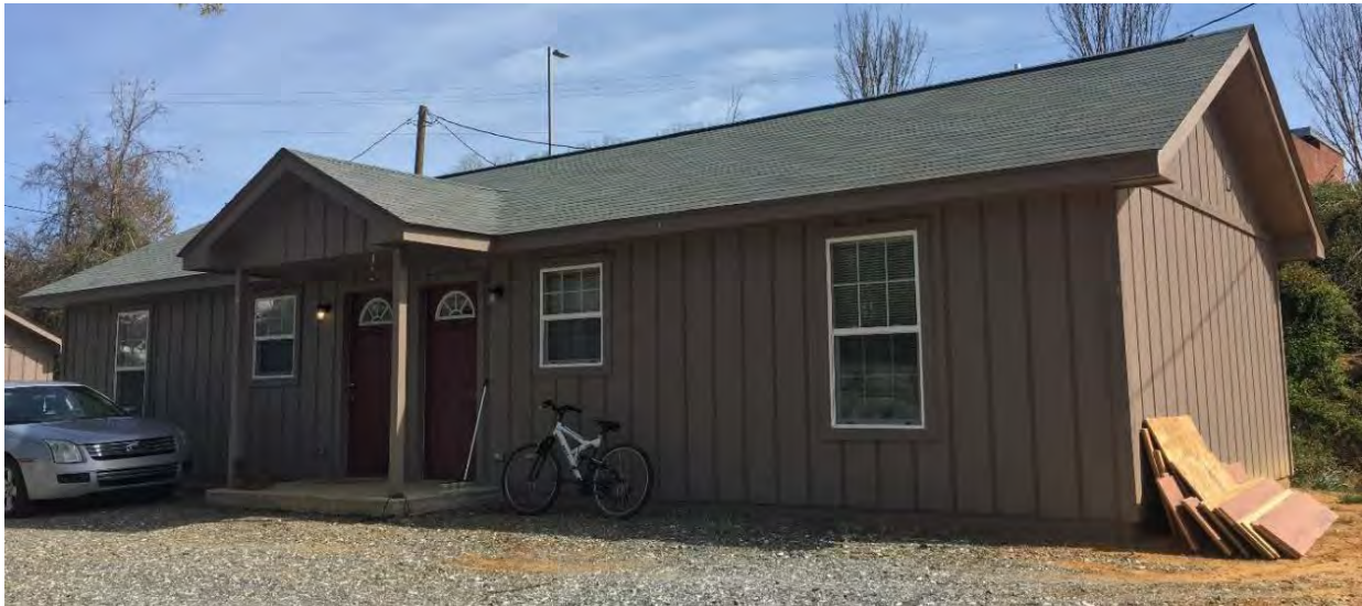
FIGURE 30: Current photo of the south elevation and façade of Duplex #2 facing south
