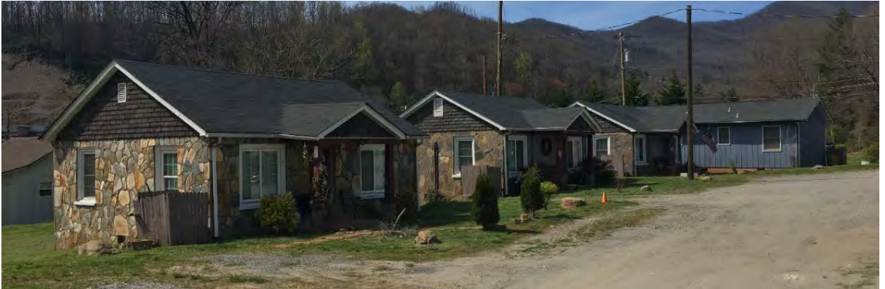
FIGURE 22: Current photo of the façade of the #15, #14, and #13 cottages and rear of the triplex facing northwest
