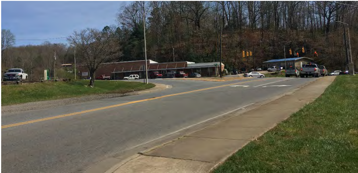
FIGURE 9: View from the southeast corner of the property towards the intersection of NC 107 and Skyland Drive, facing south
