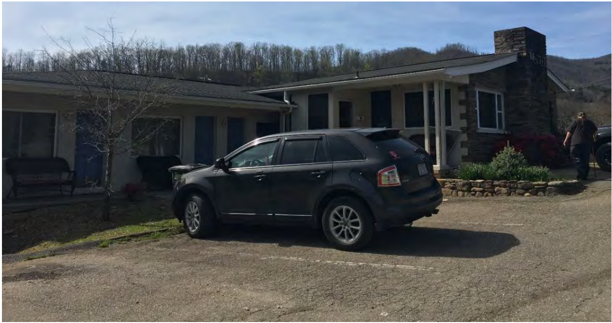
FIGURE 3: Azalea Motel (JK0104), 97 Skyland Drive, oblique front view to the northwest
