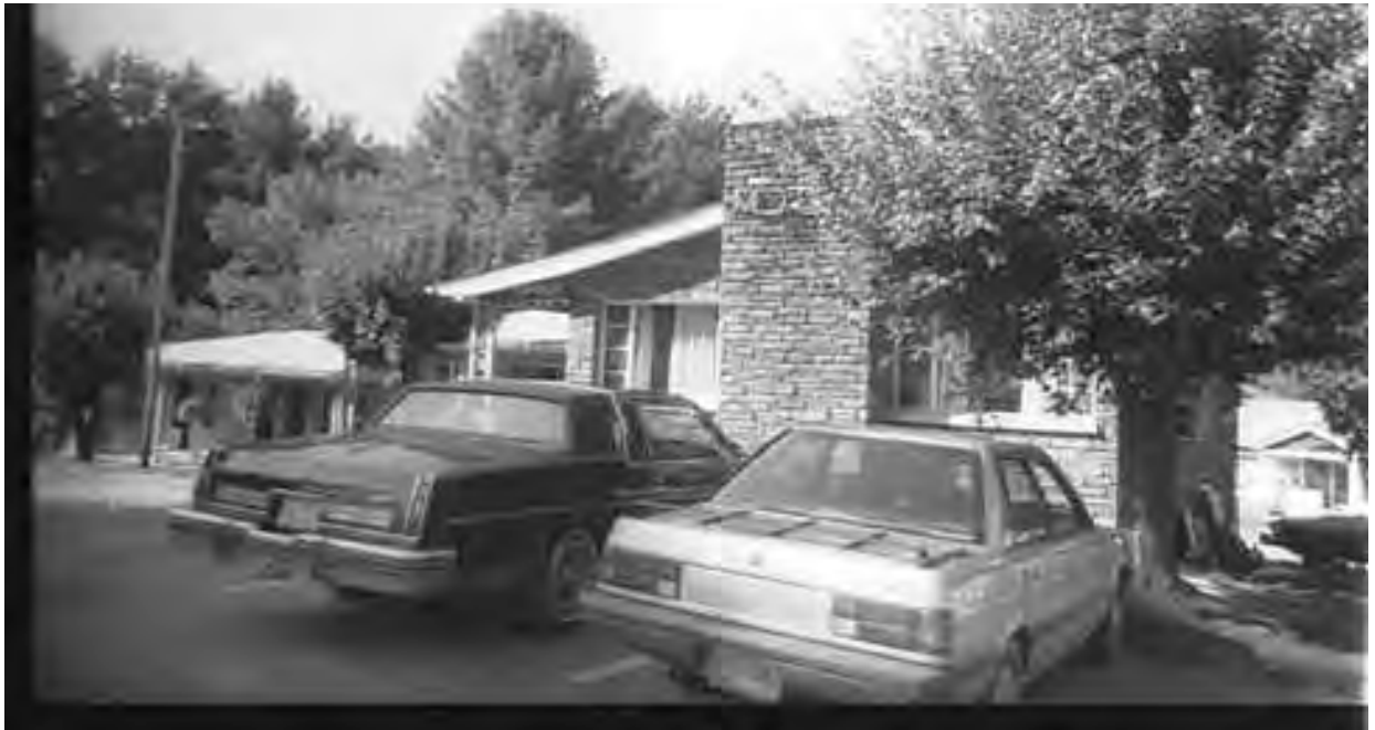
FIGURE 14: 1989 survey photo of the east façade of the office facing southwest
