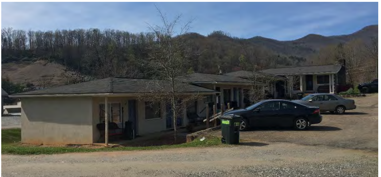
FIGURE 16: Current photo of the east façade of the motel facing northwest
